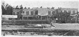
A view of the new ISI Administrative-cum-Testing Laboratory Building at Bangalore
