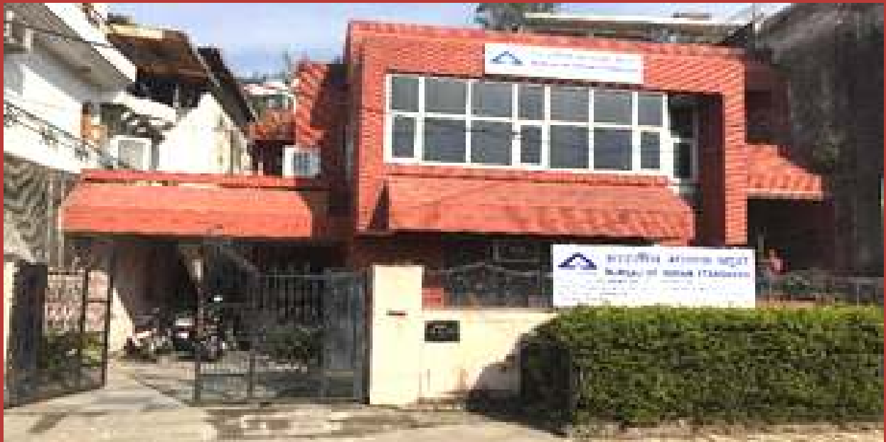
Himachal Pradesh Branch Office Parwanoo at Nalagarh Estt. 2001-02
