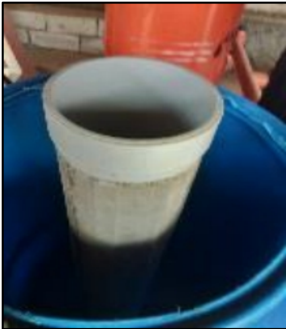
Fig 1 : Strainer inside tank
