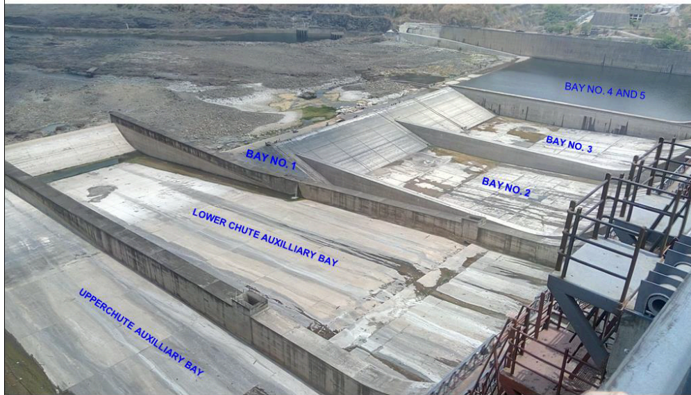
VIEW SHOWING STILLING BASIN - BAYS NO.1 TO 5
