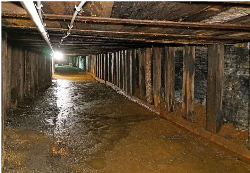
Fig.2.1. Bord and Pillar Mining (Underground)
